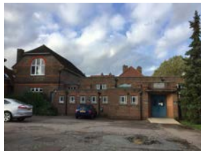
The car park
