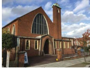
The Cranley Gardens entrance
